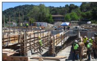
Performing Arts Building Wall Forming
