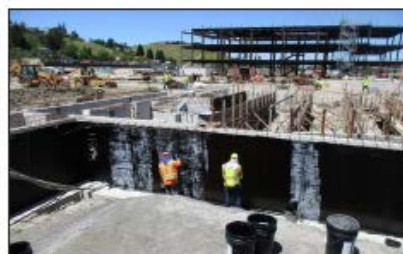
Performing Arts Building Waterproofing
